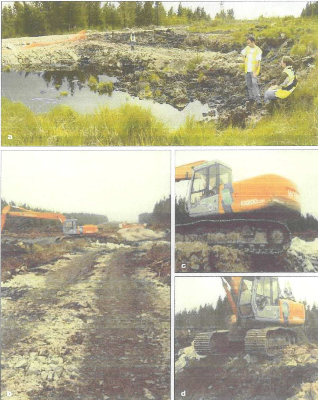
Plate 8.2: The head of the peat slide at T68. a: turbine base excavation in June 2004; b: deformation of floating road October 2003; c, d: an excavator after the bog slide.
