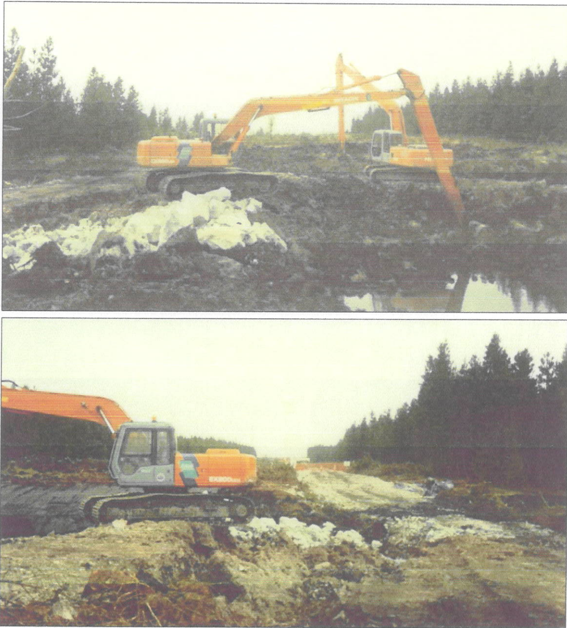
Plate 8.9: T68 shortly after the bog slide. The head of the failure was marked by a tension crack which can be seen beneath the perched excavator and the access road bowed downslope (to the right of the lower picture, which was taken from the west side of the slide).
